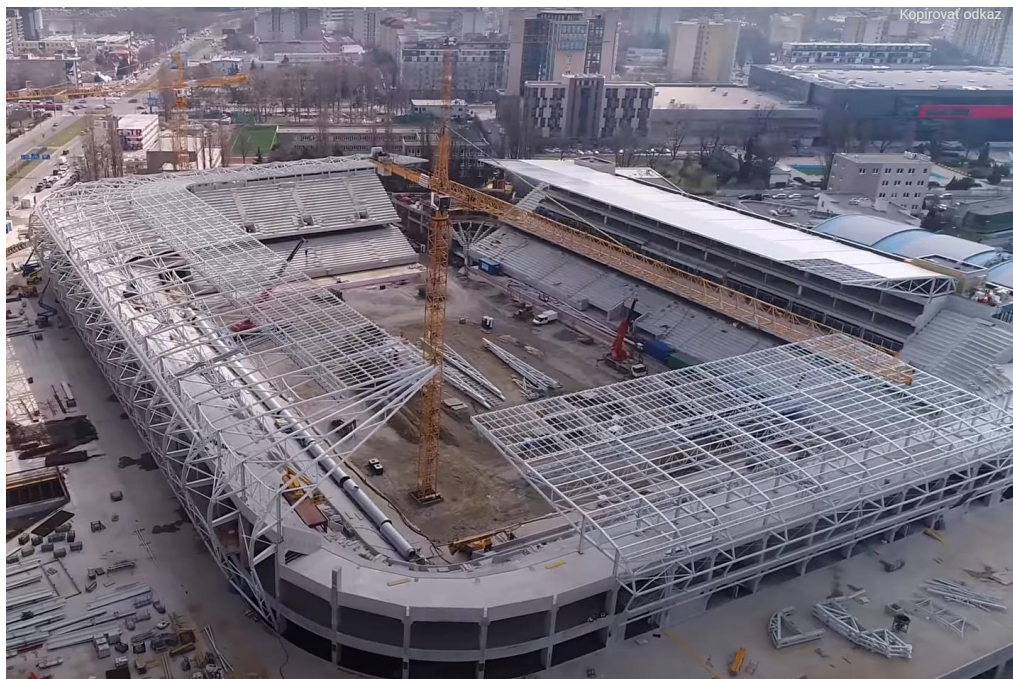
Fig. 9 Instalation of the steel structure of the grandstand roof.
