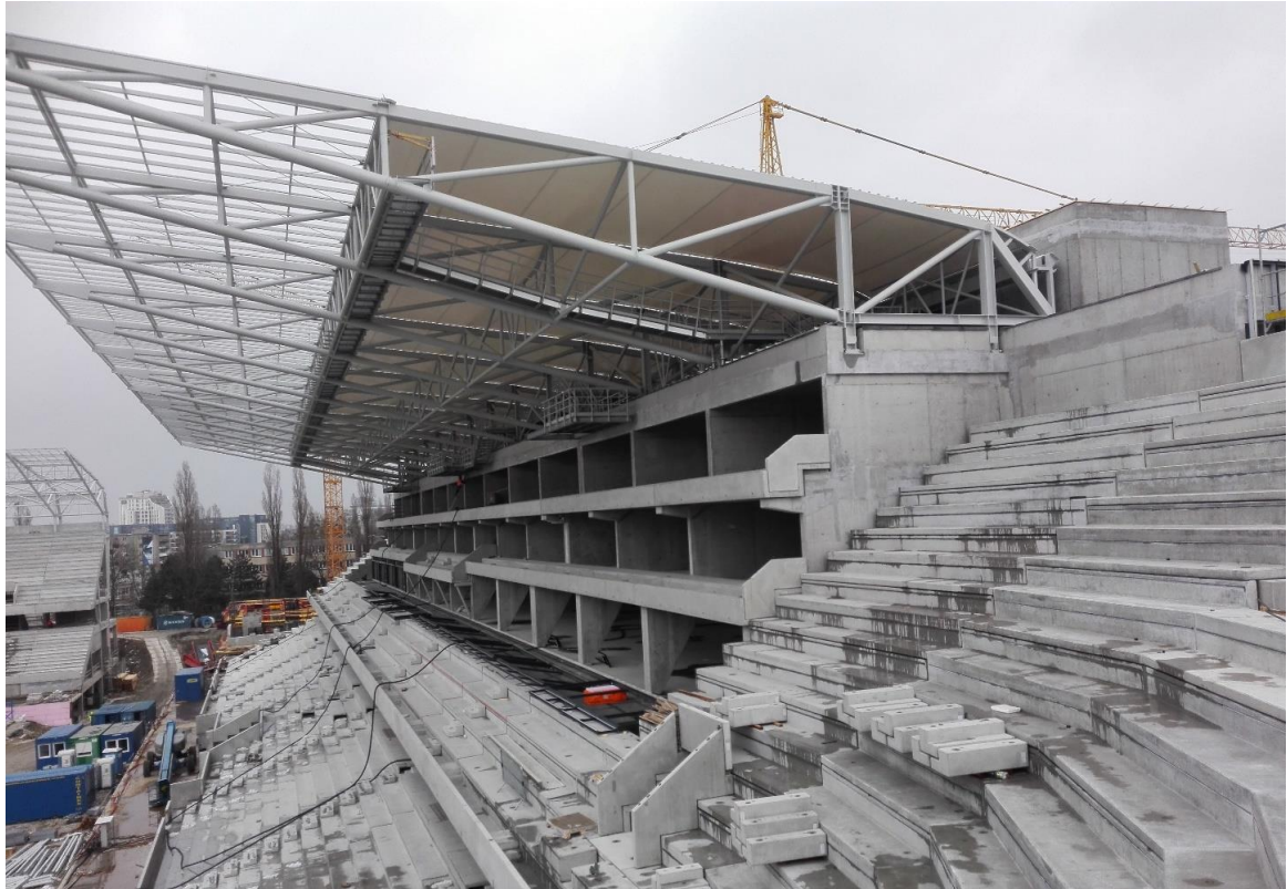
Fig. 7 Assembly of the structure of the western tribune and tribune benches.
